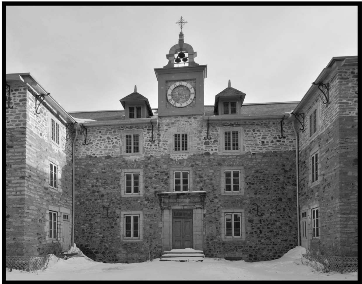
Vieux séminaire du Saint-Sulpice, 130 rue Notre-Dame ouest. The central block and stair towers were built to plans by Sulpician Superior François Dollier de Casson in 1684–87. The wings (not shown) were built to plans by Sulpician Superior François Vachon de Belmont in 1704–15.
