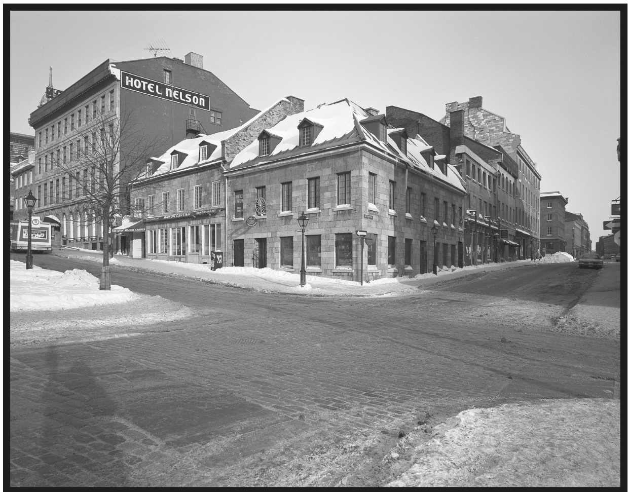
Maison Parthenais-Perrault, at the corner of Place Jacques-Cartier and rue Saint-Paul, for which Amable Amiot dit Villeneuve served as mason, 1812–13. The window openings were enlarged in 1842 to promote commerce. The ashlar façades on rue Saint-Paul were added in 1846 by mason contractor Augustin Laberge for owner Augustin Perrault.
