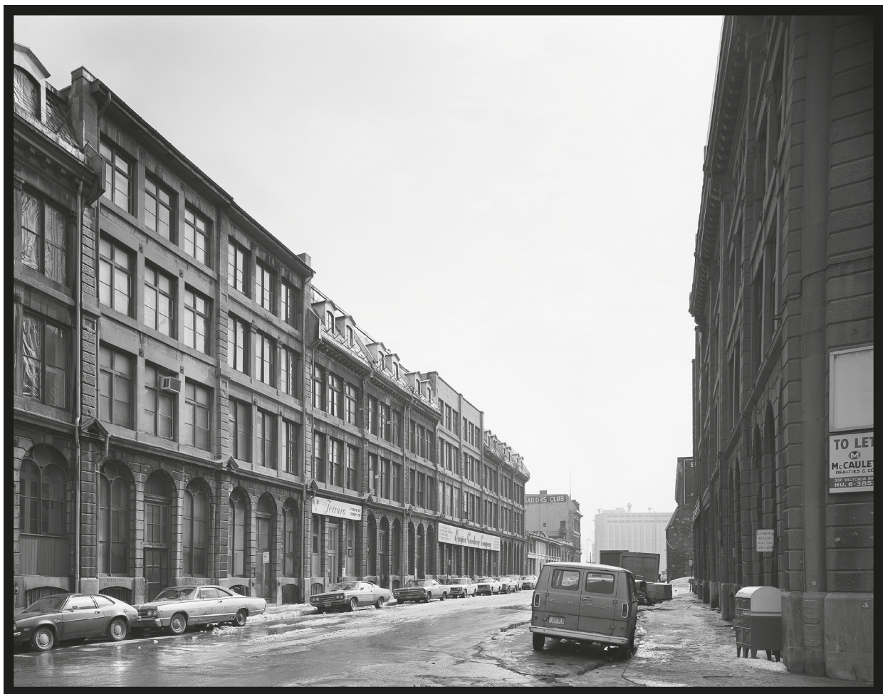
Sœurs Grises Warehouses, view south, rue Saint-Pierre (Michel Laurent, architect, built in 1872–73).
